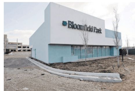
Fallen signs and unfinished buildings mark the scene of what had been planned as an 18-building, $350 million mixed-use development on the border of Pontiac and Bloomfield Township.
